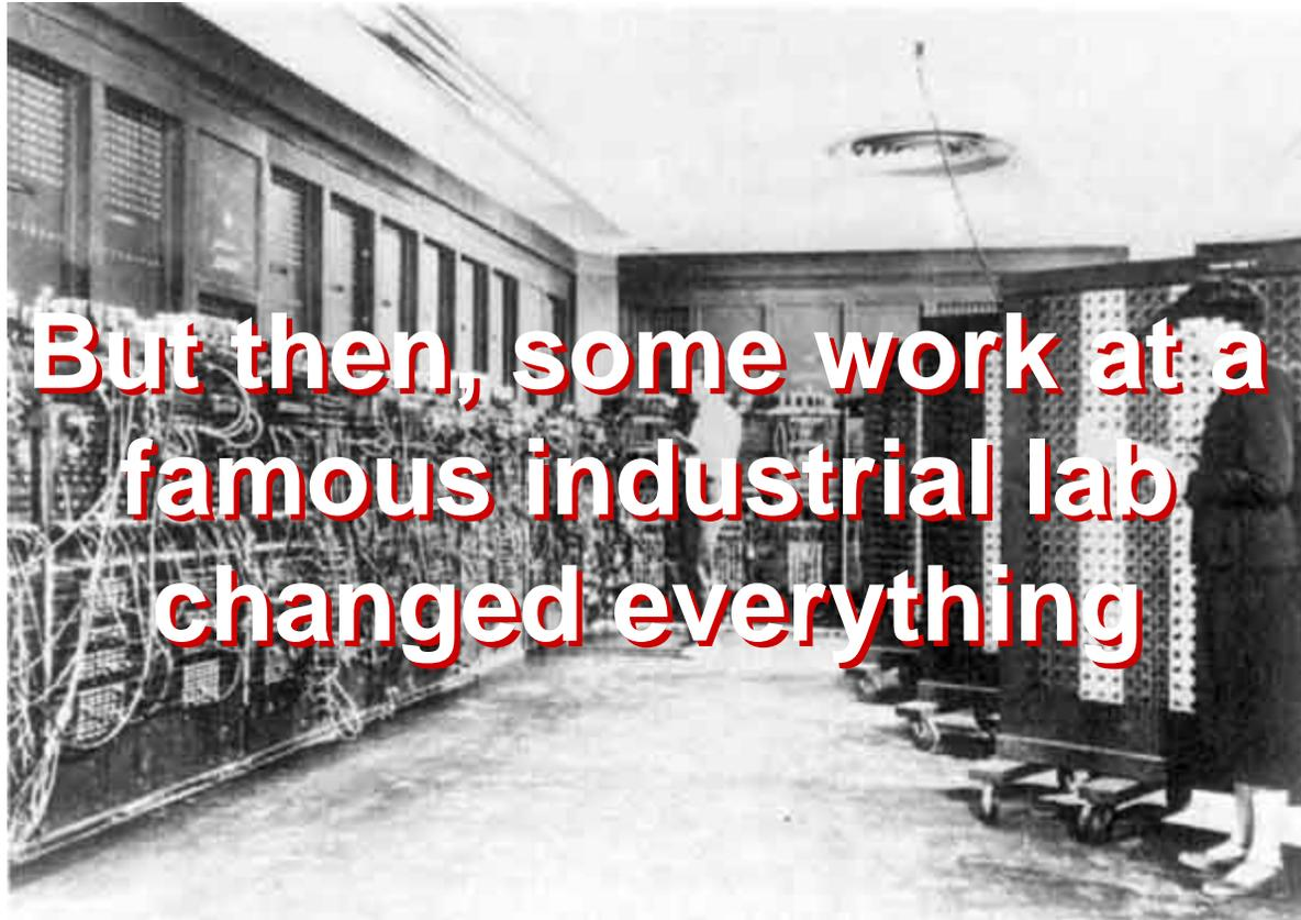
*Its thirty separate units, plus power supply and forced-air cooling, weighed over thirty tons. Its 19,000 vacuum tubes, 1,500 relays, and hundreds of thousands of resistors, capacitors, and inductors consumed almost 200 kilowatts of electrical power.*
